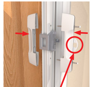
Lock Mechanism
